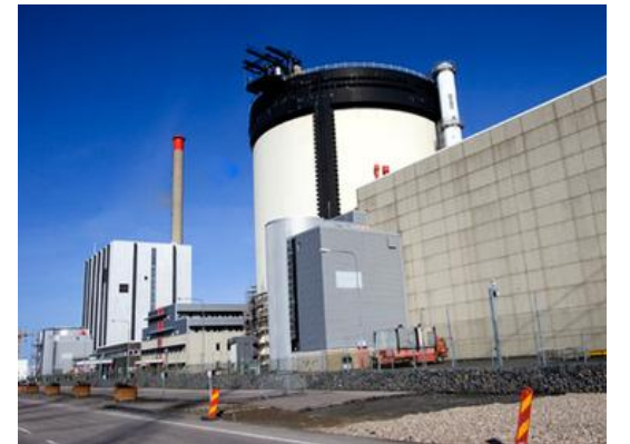
Ringhals TR3 Reactor
